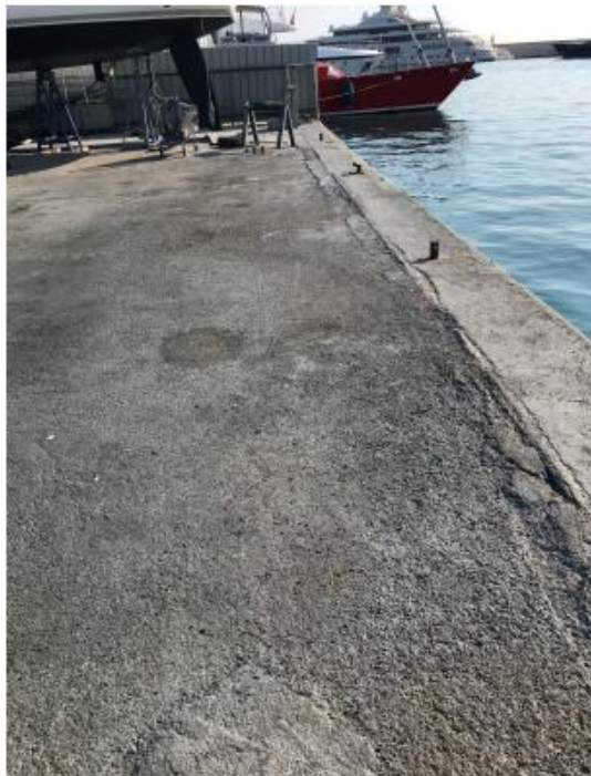
Figure 5: quai chantier naval
